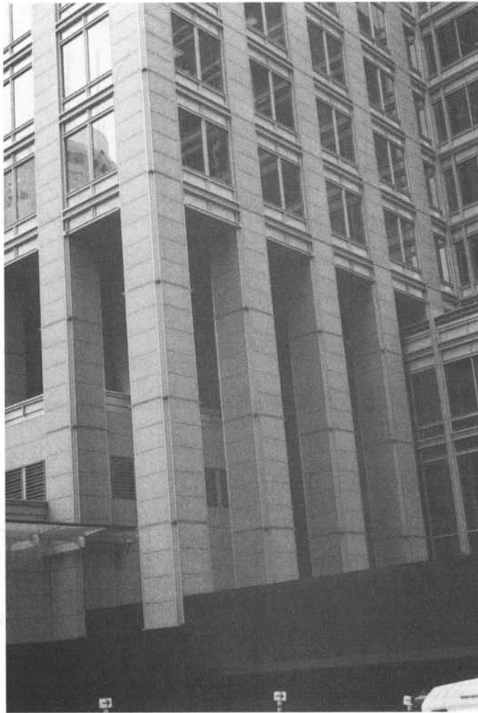
Long columns in an office building.
