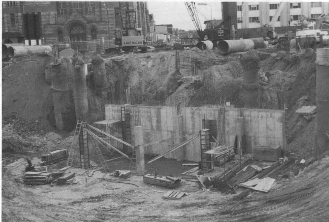
Wall and column footings, partly covered.
