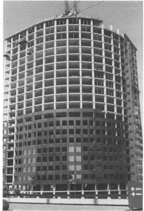
Office building under construction, New Orleans, Louisiana.
