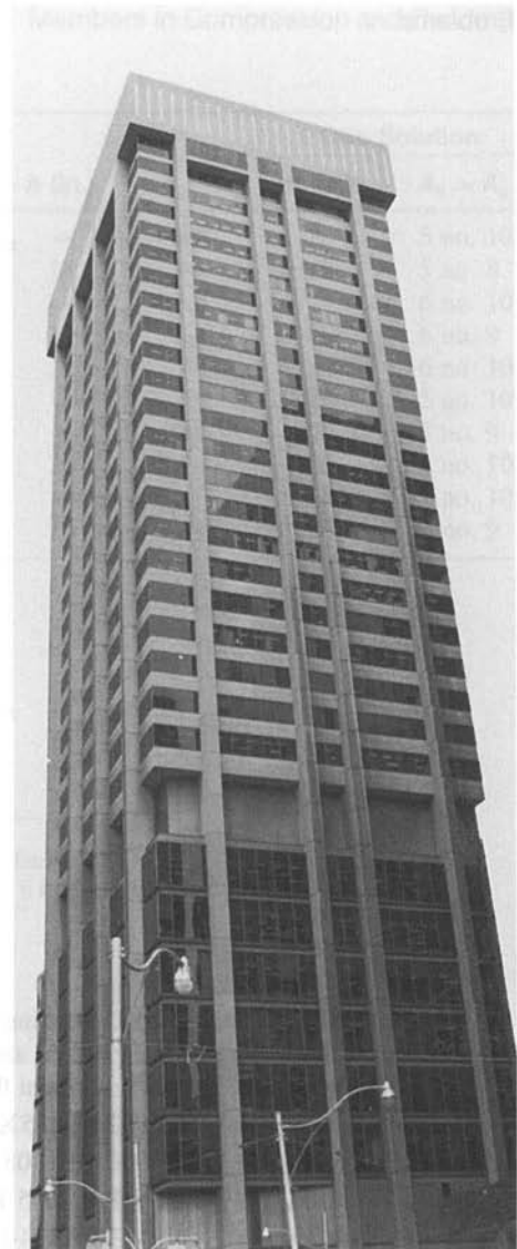
Columns in a high-rise building, Toronto, Canada.
