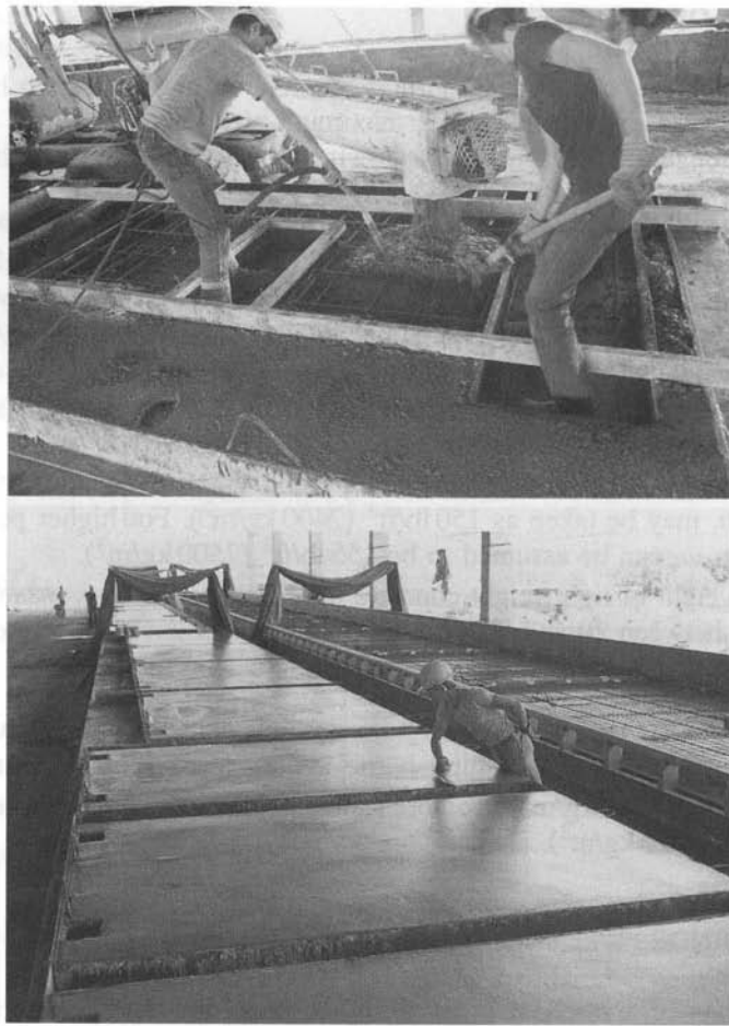
Casting and finishing precast concrete wall panels.
