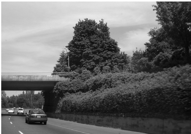
FIGURE 3.26 Well-integrated landscaping at a bridge over I-5 in Olympia, Washington.
