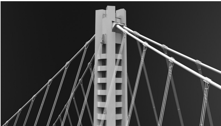
FIGURE 1.26 The new SFOBB tower configuration.
