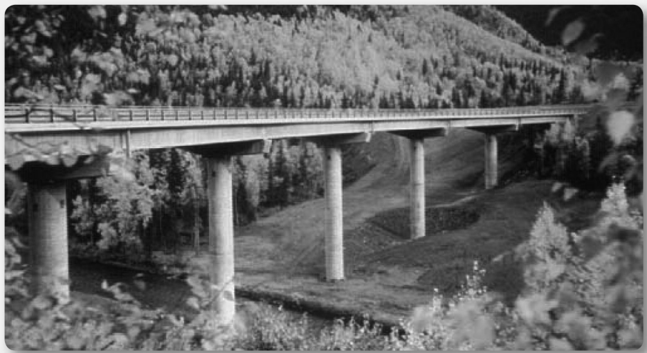
FIGURE 3.1 Often simply paying attention to proportions and details can result in an attractive bridge with no increase in cost. Canyon Creek Bridge, Anchorage, Alaska. (From AASHTO, Bridge Aesthetics Sourcebook , American Association of State Highway and Transportation Officials, Washington, DC, 2010. With permission.)
