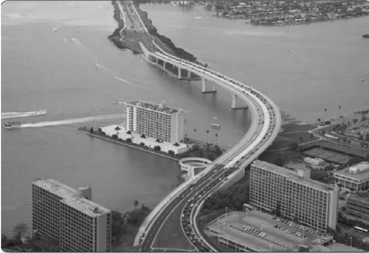
FIGURE 3.16 An example of a successful collaboration between an engineer and an architect/urban designer which considers nearby land uses and views as well as technical requirements. Clearwater Memorial Causeway, Clearwater, Florida. (From AASHTO, Bridge Aesthetics Sourcebook , American Association of State Highway and Transportation Officials, Washington, DC, 2010. With permission.)
