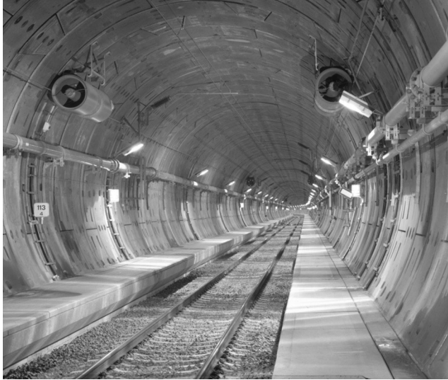
FIGURE 4.8 Great Belt, East Tunnel, Denmark. (Courtesy of Sund & Bælt Holding A/S.)
