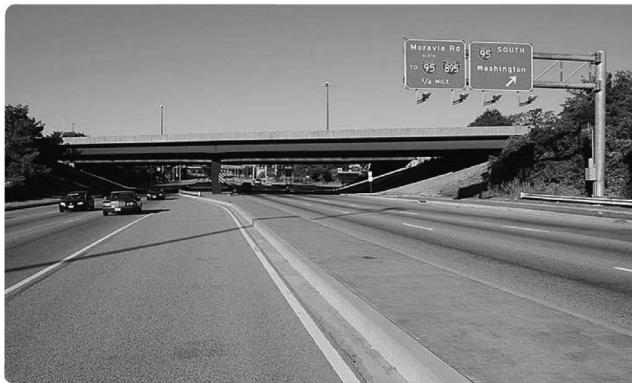
FIGURE 3.21 These minimum-height abutments essentially disappear behind the trees, maximizing the opening under the bridge and the view through to the area beyond. It is also a good example of the values to be gained by thinness and simplicity. I-95 over Pulaski Highway, Baltimore, Maryland ( Sourcebook 1–4). (From AASHTO, Bridge Aesthetics Sourcebook , American Association of State Highway and Transportation Officials, Washington, DC, 2010. With permission.)
