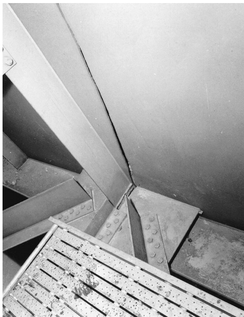
FIGURE 19.1 View of cracked girder of Lafayette Street Bridge in Minneapolis showing fatigue crack originating from backing bars and lack of fusion on the weld attaching the lateral bracing attachment plate to the web and to the transverse stiffener.
