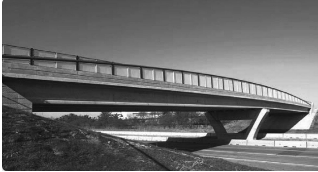
FIGURE 3.22 This pedestrian fence uses standard chain link, but the arched top edge, carefully designed details and distinctive color improve the appearance of the bridge without a significant increase in cost, I-235 Reconstruction, Des Moines, Iowa ( Sourcebook 4–24). (From AASHTO, Bridge Aesthetics Sourcebook , American Association of State Highway and Transportation Officials, Washington, DC, 2010. With permission.)
