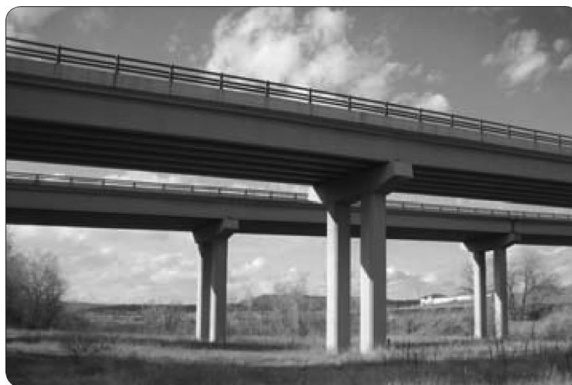
FIGURE 3.19 The substructure for this high-level crossing with slender piers is virtually transparent. Meadows Parkway over Plum Creek, Castle Rock, Colorado (Sourcebook 3.6). (From AASHTO, Bridge Aesthetics Sourcebook , American Association of State Highway and Transportation Officials, Washington, DC, 2010. With permission.)
