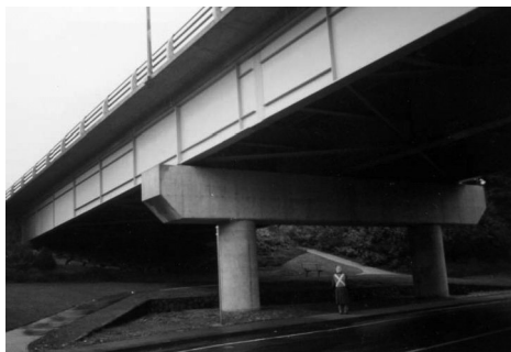
FIGURE 16.14 Rehabilitated columns of the Portage Creek Bridge in British Columbia, Canada.
