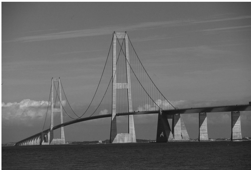
FIGURE 4.6 Great Belt, East Bridge, Denmark. (Courtesy of Sund & Bælt Holding A/S.)
