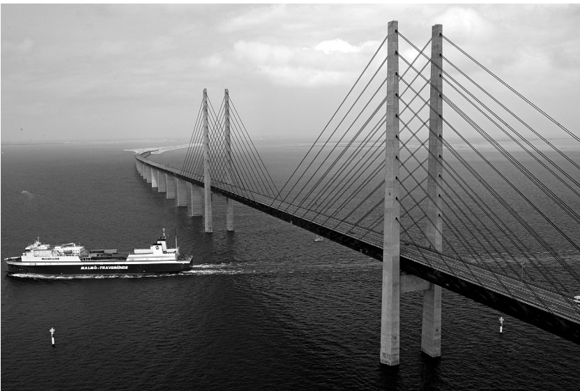
FIGURE 4.9 Øresund Link, cable-stayed bridge, Denmark–Sweden. (Courtesy of Søren Madsen/Øresundsbron.)
