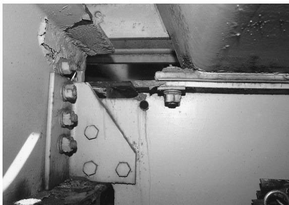
FIGURE 19.6 View of floorbeam of Throg's Neck Bridge in New York showing crack in the cope that has been repaired by drilling a stop hole. The crack is caused by incompatibility between the curvature of the superstructure and the orthotropic steel deck that is bolted onto the floorbeams.
