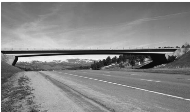
FIGURE 3.13 Genesee Mountain Interchange, I-70, Colorado. As motorists travel west from Denver on I-70, this bridge frames their first view of the Rocky Mountain peaks along the Continental Divide. (From AASHTO 2010, Bridge Aesthetics Sourcebook , American Association of State Highway and Transportation Officials, Washington, DC, 2010. With permission.)
