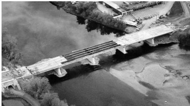
FIGURE 16.21 Aerial view of Joffre Bridge during construction. (From ISIS, Design Manual 3: Reinforcing Concrete Structures with Fibre Reinforced Polymers . ISIS Canada, Intelligent Sensing for Innovative Structures, A Canadian Network of Centres of Excellence, University of Manitoba, Winnipeg, Manitoba, Canada, 2007a. With permission.)
