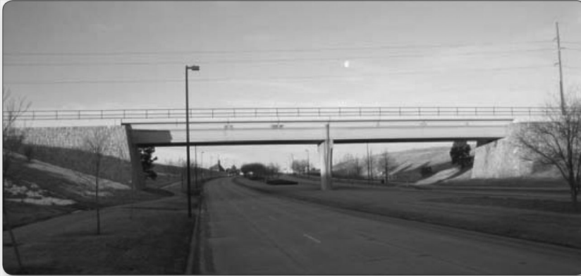
FIGURE 3.20 This full-height abutment frames a portion of the landscape beyond the bridge. Meadows Parkway Railroad Overpass, Castle Rock, Colorado ( Sourcebook 2.8). (From AASHTO, Bridge Aesthetics Sourcebook , American Association of State Highway and Transportation Officials, Washington, DC, 2010. With permission.)
