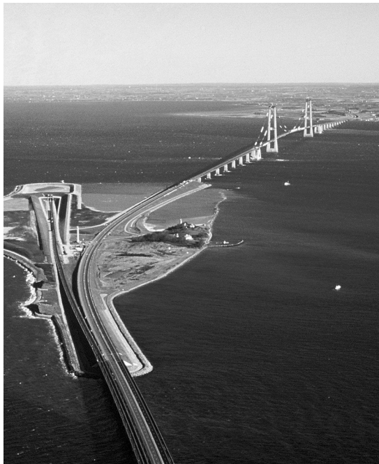
FIGURE 4.5 The Great Belt Fixed Link. Combined road and rail low-level West Bridge in foreground, East Bridge suspension road bridge, and ramp to the East Tunnel for railway. (Courtesy of Sund & Bælt Holding A/S.)
