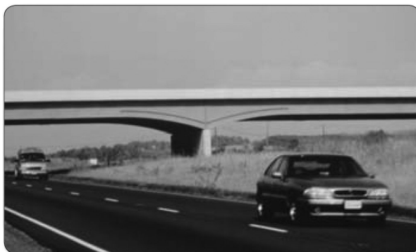
FIGURE 3.18 The haunch gives this girder a more interesting and attractive shape that also tells a story about the flow of moments and forces in the structure. The stiffener is utilitarian but its placement and curvature make it ornamental as well, so that it reinforces the story told by the haunch. I-81, Virginia. (From AASHTO, Bridge Aesthetics Sourcebook , American Association of State Highway and Transportation Officials, Washington, DC, 2010. With permission.)
