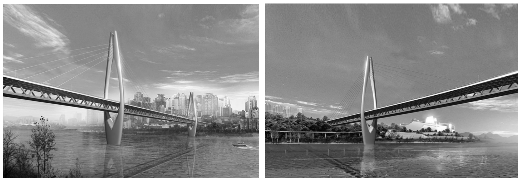
FIGURE 1.23 The Twin River Bridge—Dongshuimen Bridge and Qianshimen Bridge.
