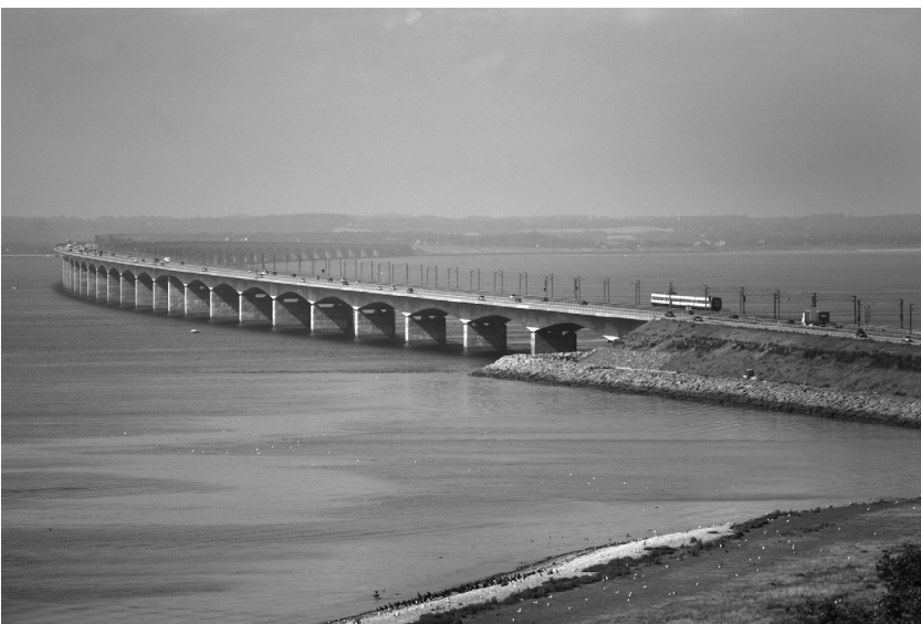
FIGURE 4.7 Great Belt, West Bridge, Denmark. (Courtesy of Sund & Bælt Holding A/S.)
