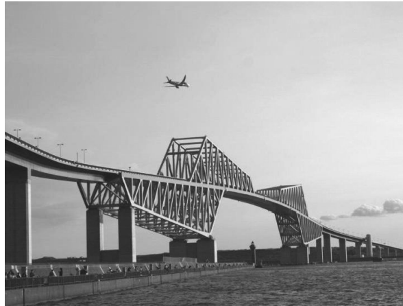
FIGURE 17.2 Tokyo Gate Bridge.
