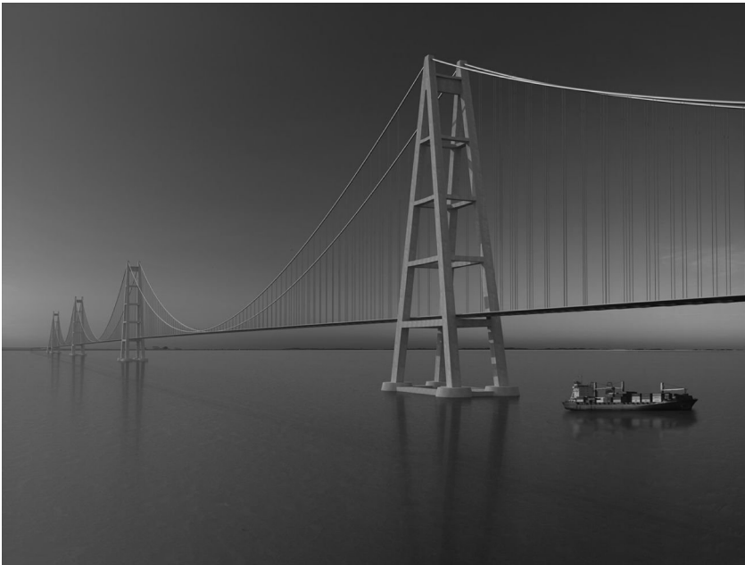
FIGURE 4.1 Rendering of the proposed multi-span suspension bridge connecting Yemen and Djibouti. (Courtesy of Dissing+Weitling architecture.)
