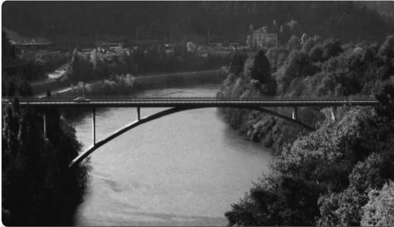
FIGURE 3.6 Rock foundations permit arch bridges. Christian Menn's Reichenau Bridge, Switzerland. (From AASHTO, Bridge Aesthetics Sourcebook , American Association of State Highway and Transportation Officials, Washington, DC, 2010. With permission.)
