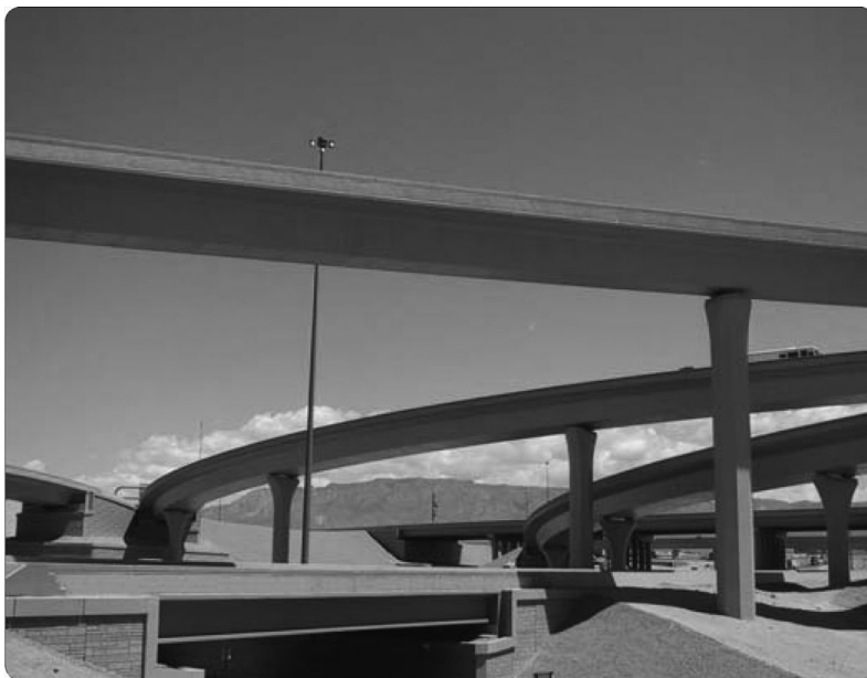
FIGURE 3.14 Albuquerque's Big I interchange has a theme covering pier shapes, MSE walls, standard details, and colors, the latter developed with community input. (From AASHTO, Bridge Aesthetics Sourcebook , American Association of State Highway and Transportation Officials, Washington, DC, 2010. With permission.)
