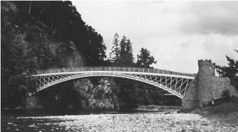
FIGURE 3.4 Thomas Telford's Craigellachie Bridge.
