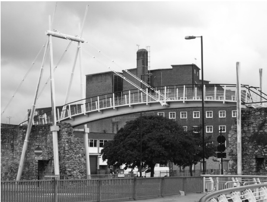
Figure 1.9 A footbridge with cable stayed mid-span support, Southampton, UK.
