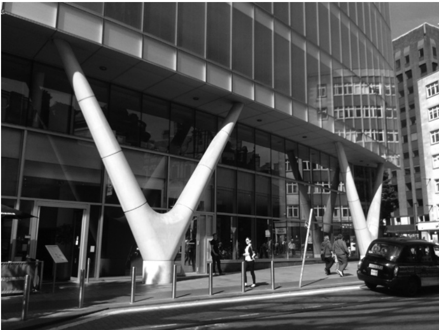
Figure 6.21 Variable cross-section of the arms of Y shaped columns in a building, UK.
