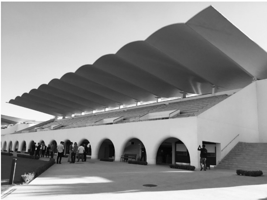
Figure 4.23 A front view of the Madrid Racecourse Stand, Spain.
