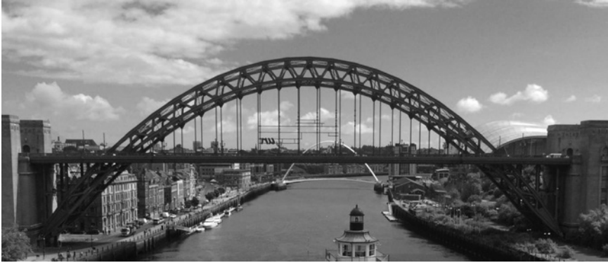
Figure 5.18 The Tyne Bridge in Newcastle upon Tyne, UK.
