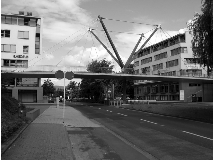
Figure 4.19 Hessenring Footbridge, Bad Homberg, Germany (Courtesy of Mr. Per Waahlin, Sweden).
