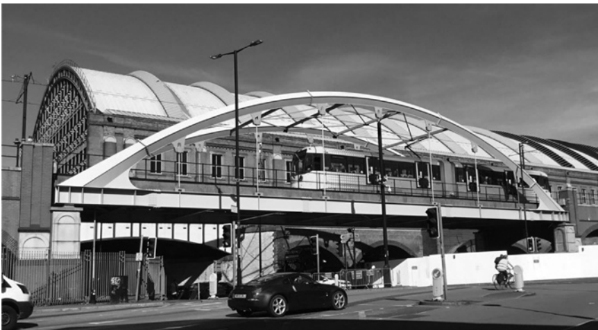
Figure 4.27 The arch, deck and cables of the bridge form a self-balancing system.
