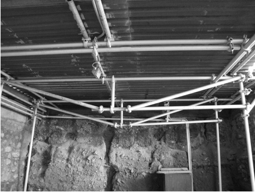
Figure 2.8 Additional supports to a floor.
