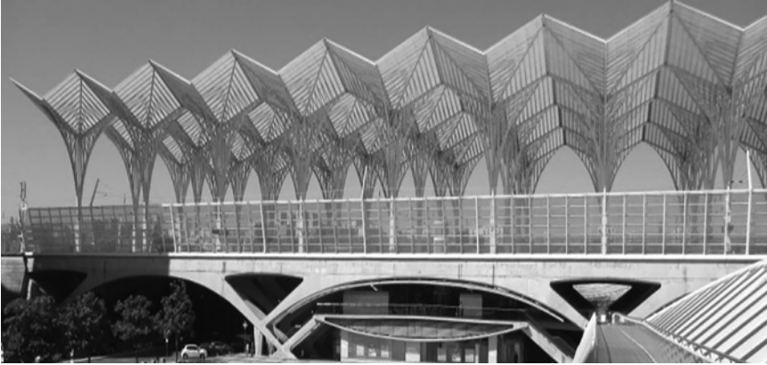
Figure 4.20 A tree-like structure as an evolution of a series of Y shaped columns.
