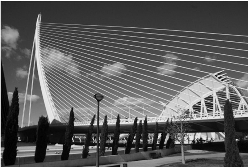
Figure 5.7 The Serreria Bridge, Valencia, Spain (Courtesy of Mr. Nicolas Janberg, structurae.net , Germany).
