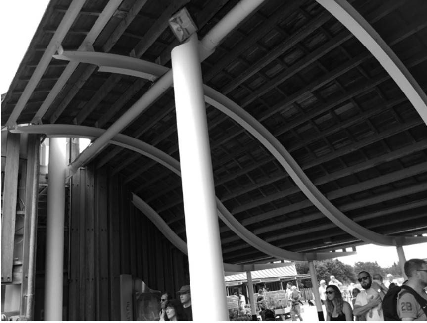
Figure 4.4 Simply supported curved beams with overhangs.
