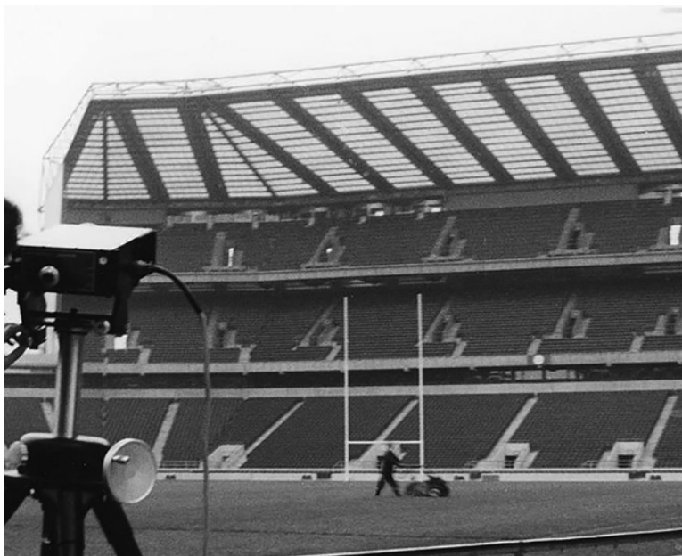
Figure 1.6 The North Stand, Twickenham.
