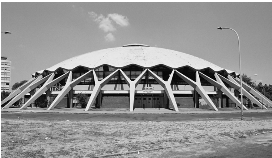
Figure 4.17 Outlook of the Palazzetto dello Sport (Courtesy of Mr. Nicolas Janberg, structurae.net , Germany).
