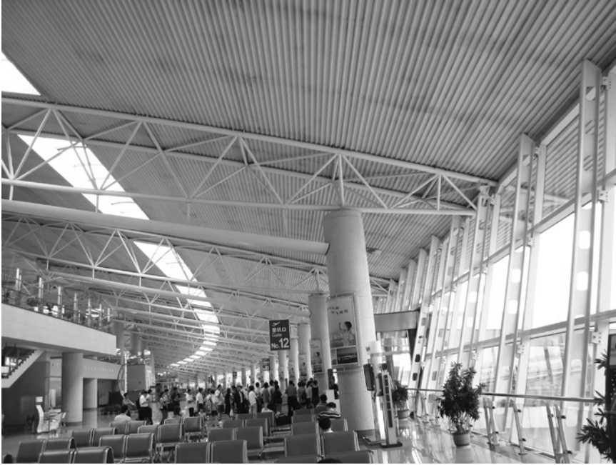
Figure 4.14 A roof structure with overhangs in an airport terminal, Harbin, China.
