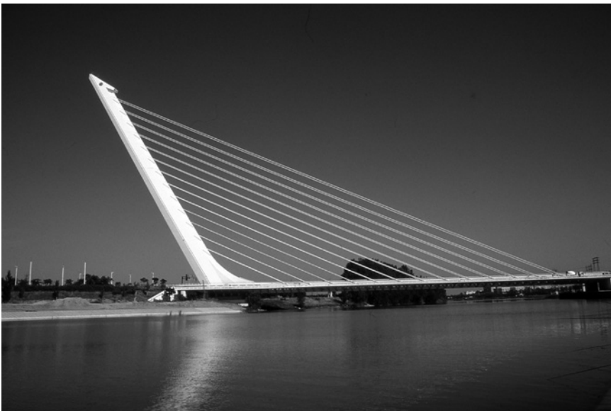
Figure 6.19 The Alamillo Bridge, Spain (Courtesy of Mr Per Waahlin, Sweden).
