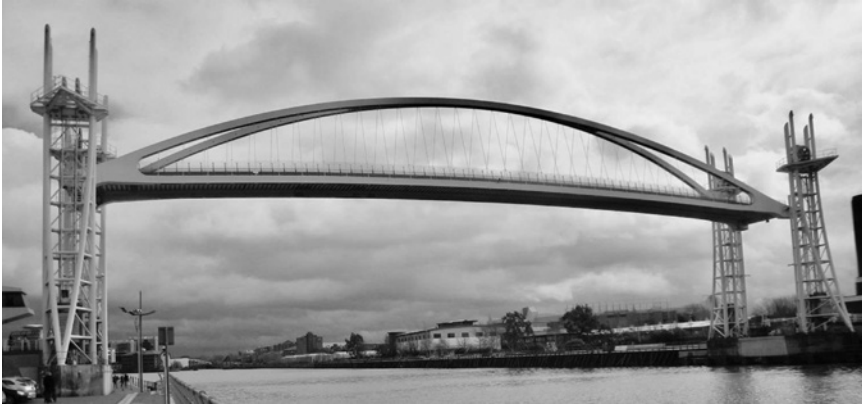
Figure 4.26 Salford Quays Lift Bridge.
