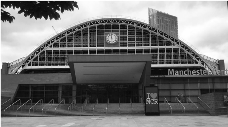
Figure 5.9 Front view of the Manchester Central Convention Complex (MCCC), Manchester.
