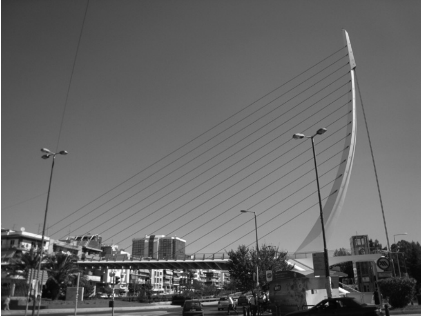
Figure 5.8 Katehaki pedestrian bridge, Athens.
