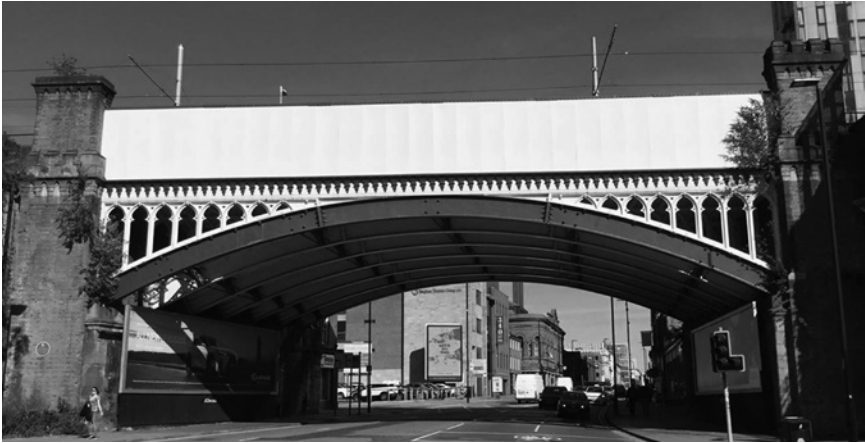
Figure 5.16 A cast iron arch bridge in Manchester.
